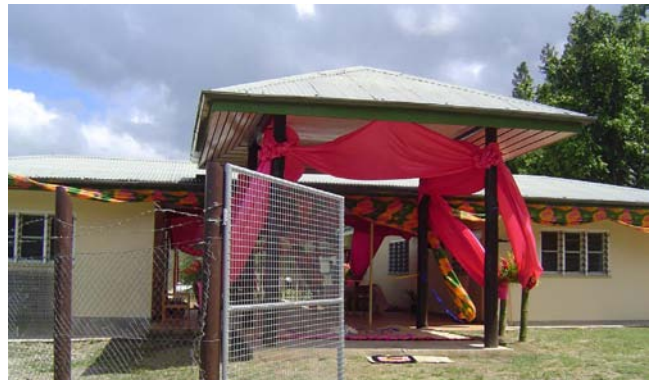
The New Nakorosule Health Centre, Naitasiri.
